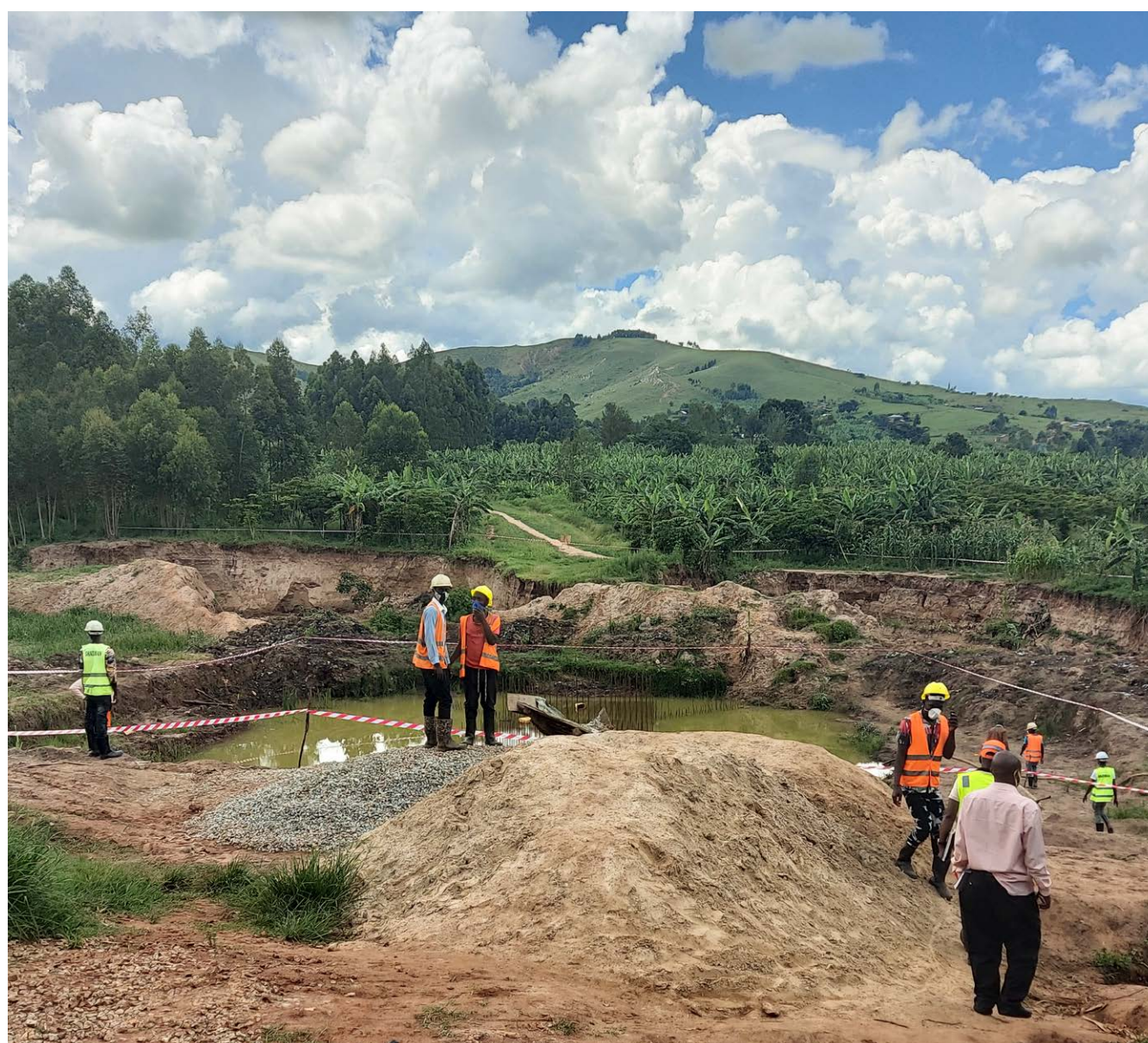
On going works in Kyenjuba Kakanena Ntungamo District
