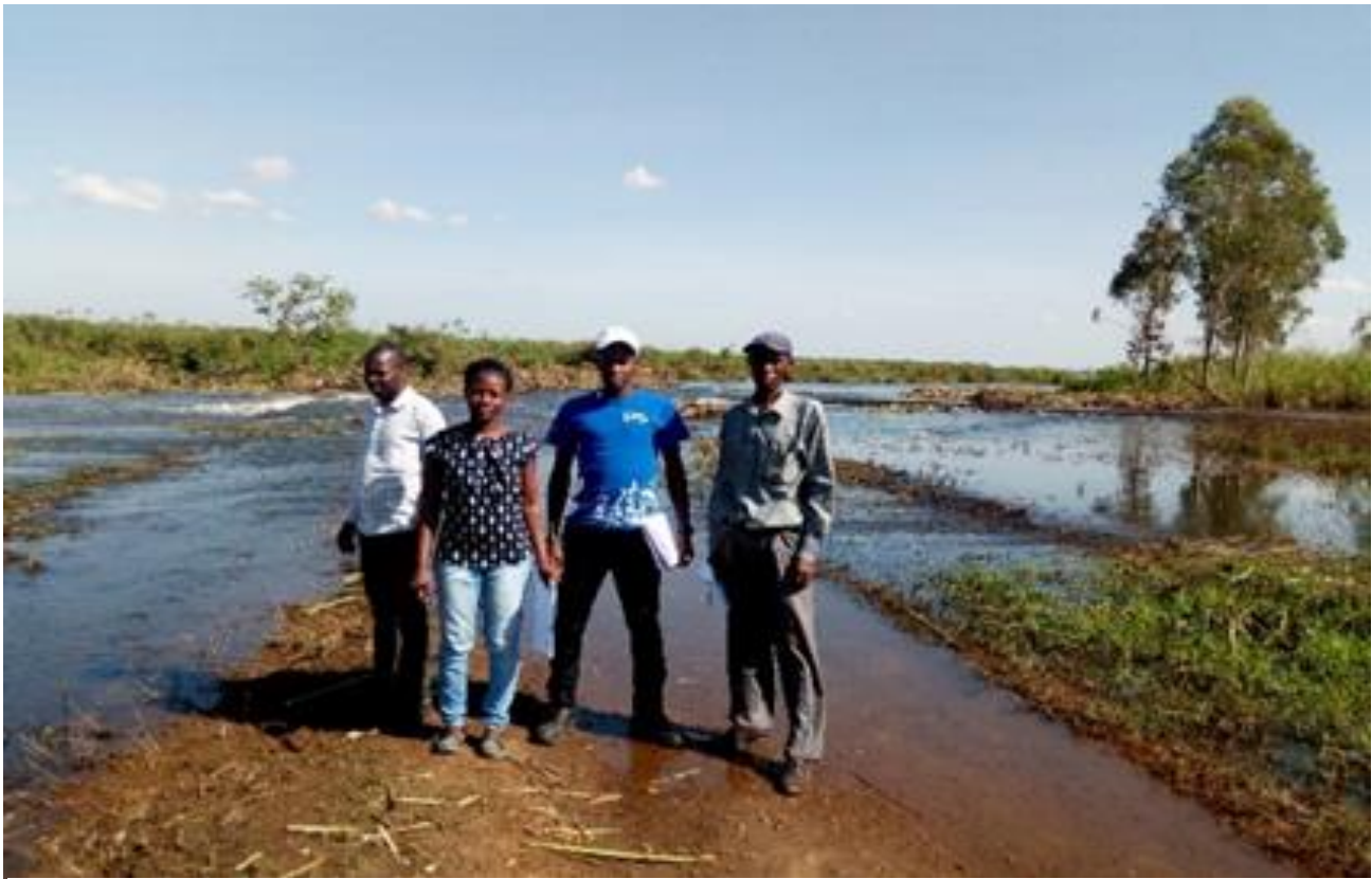
Effects of heavy rains on Nabitende -Bwengo road in Iganga Cluster
