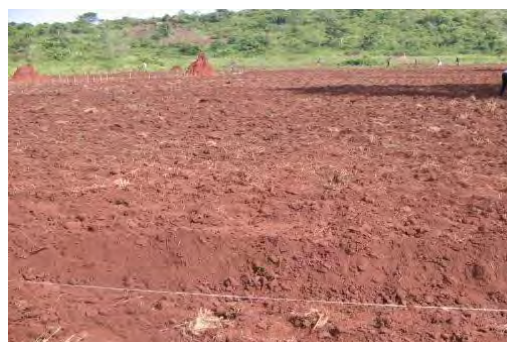
Field marking using strings
